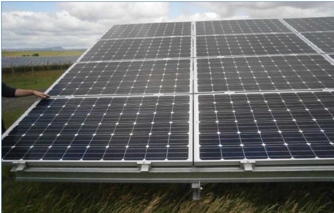
Figure 7-1 Typical Solar Panel Arrangement (showing expansion gaps)
